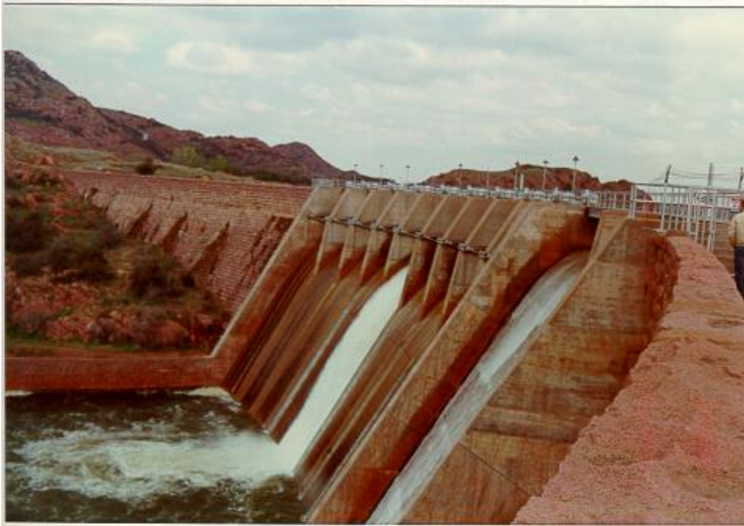
Figure 2 - Downstream Face of Altus Dam.
